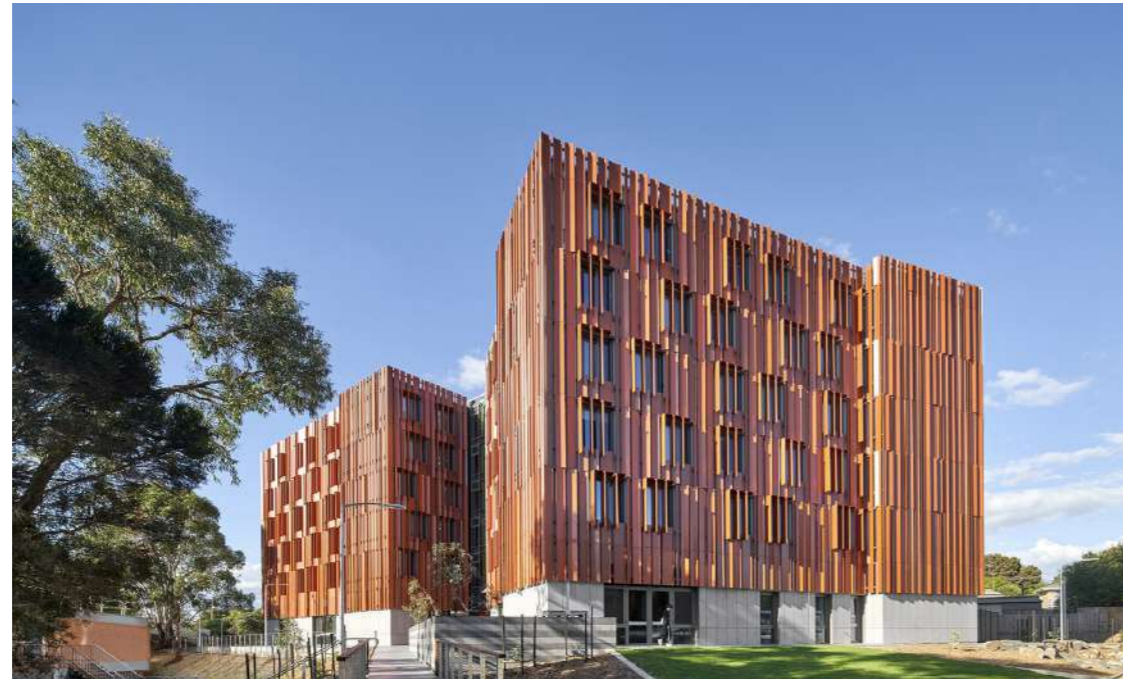
2/ 6 STOREY STUDENT HOUSING - PASSIVE HAUS + CLT TIMBER
