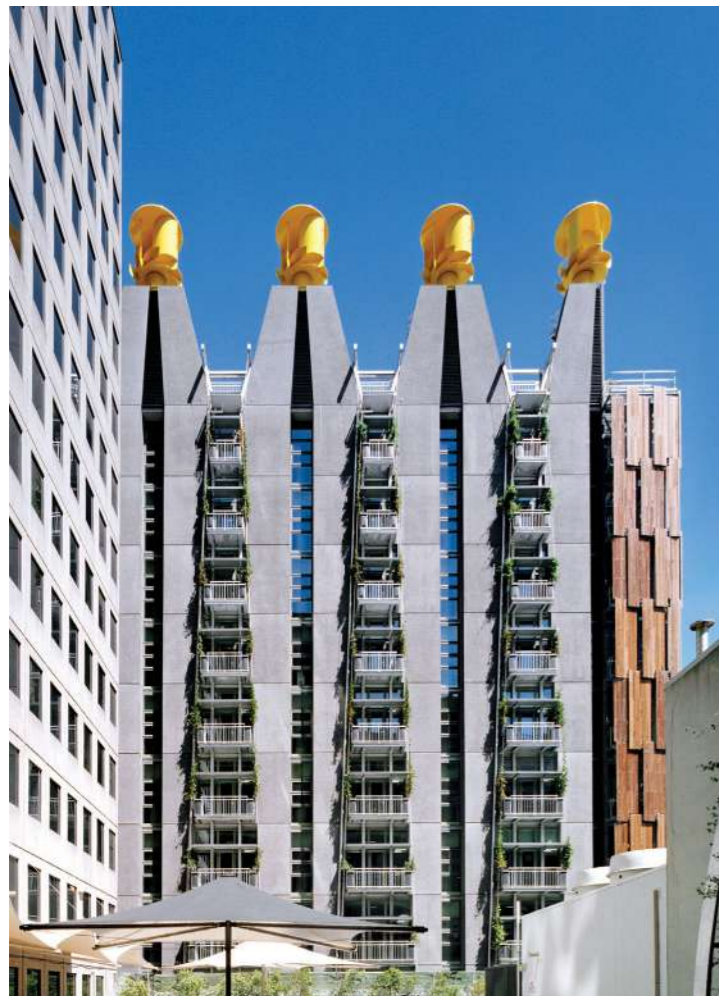
1/ WIND TURBINES - ENERGY GENERATION + ASSISTS NATURAL VENTILATION
