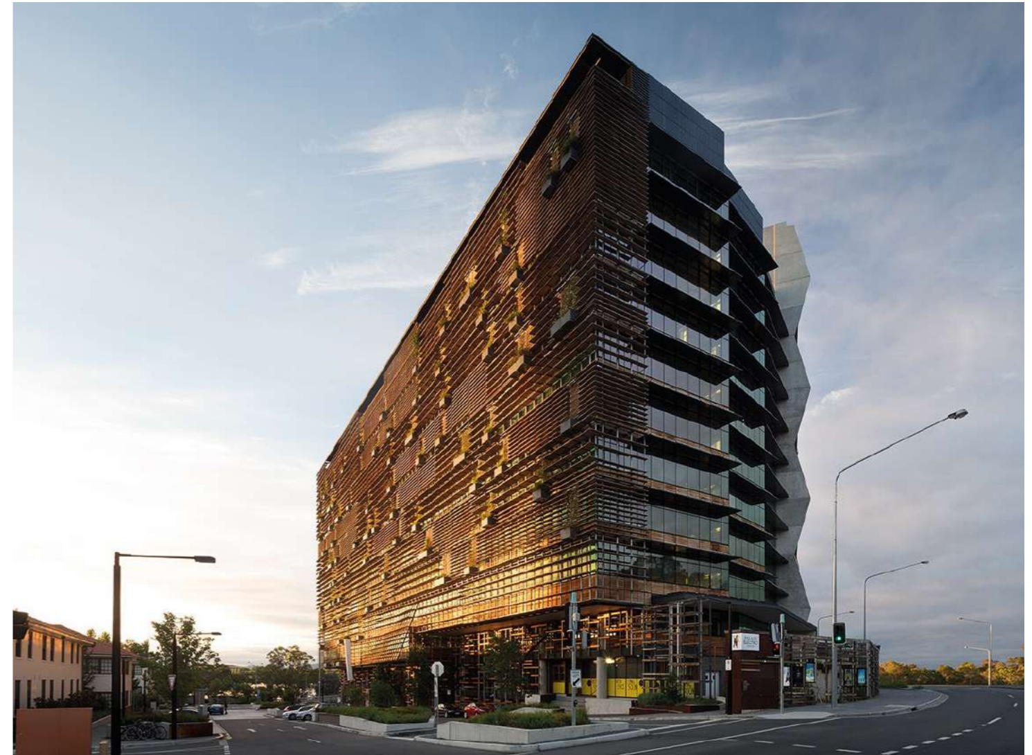
3/ FACADE SHADING - HEAT LOAD MANAGEMENT
