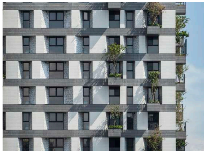
1/ HIGH SOLID TO VOID RATIO + DEEP REVEALS
