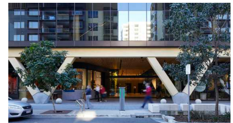
3/ GROUND LEVEL SHELTER
